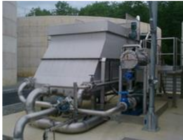
Pressurization system (dissolving tube and pump)
