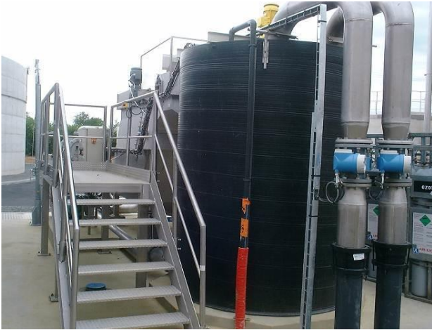
Coagulation tank Gangway to the unit
