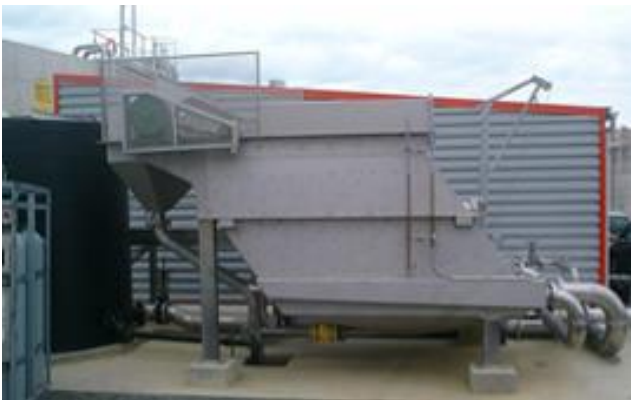
Coagulation tank Gangway to the unit
