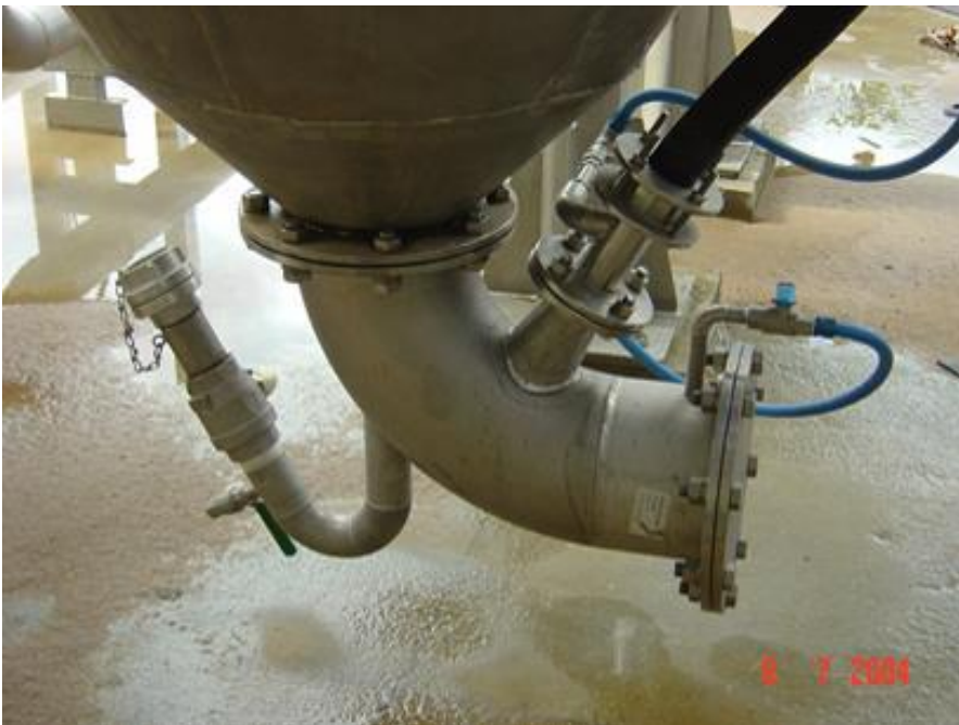
Airlift detail KS Filter air line
