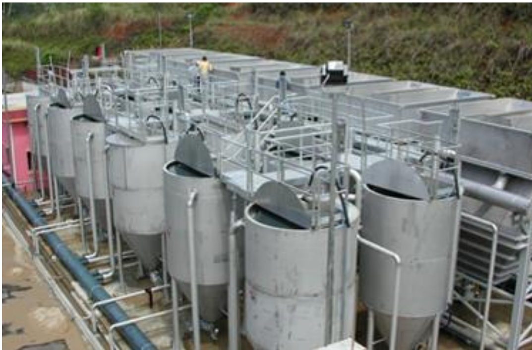
The finished installation
